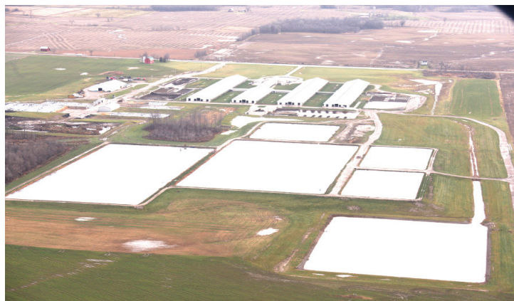
Manure lagoons at SMD 2 on US-127. None have monitoring wells or flow metering. Photo: ECCSCM/Sierra Club/Lighthawk
