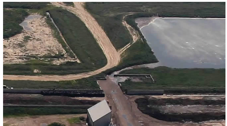
Close-up of SMD 1 "composting" area, upper left, bunker with collapsed wall, lower right.
