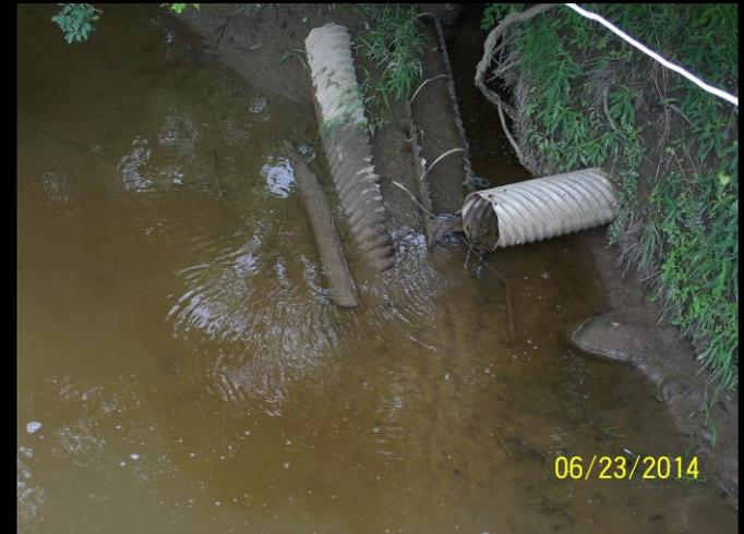
It all starts with the tiles ... 30 ft. apart, 18" or deeper, underground. Many of these private systems are unmapped. Sub-surface field tiles drain to streams.
