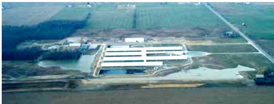
Vreba-Hoff 2 facility on US-127, nearly surrounded with contaminated stormwater (March 27, 2003)
